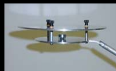
Passive Sampler installed in Ott-Peters shelter.
